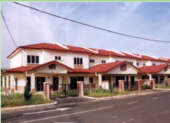
Double-storey terrace houses, ASIATIC Indahpura - Pavonina D (above) - Roseus II (below)
