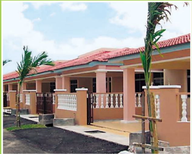
Asiatic Cheng Perdana - completed units of double- and single-storey terrace houses
