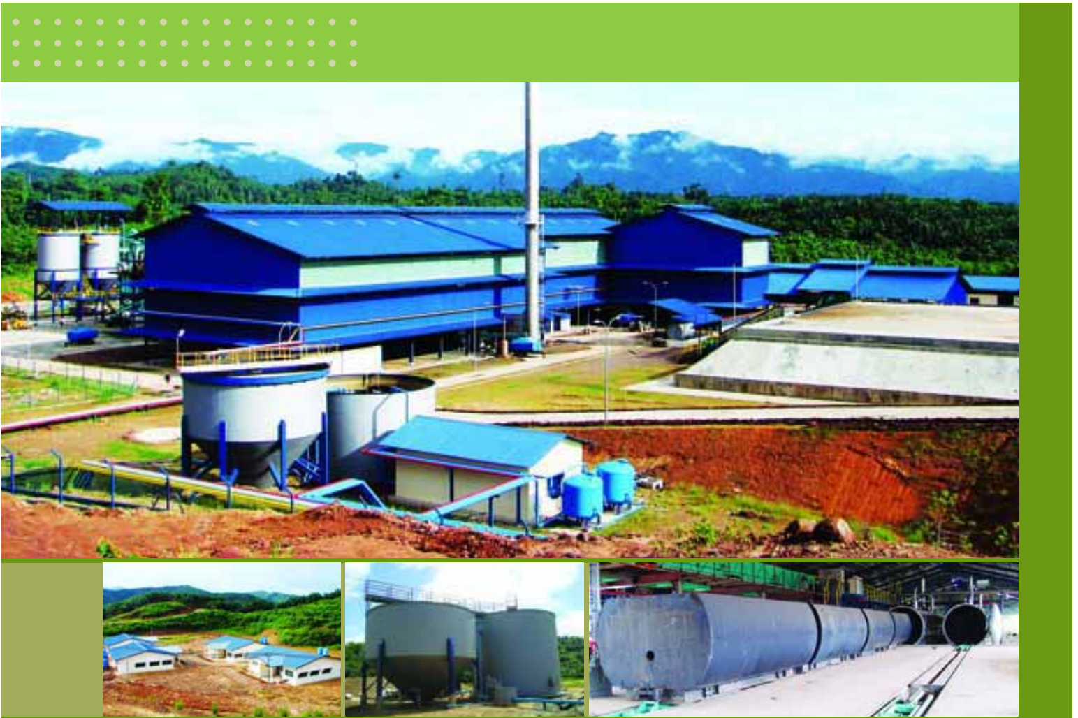
Asiatic Indah Oil Mill, Sabah - (clockwise) overview, 15 metric tonne FFB cages, advance waste water treatment plant, staff quarters
