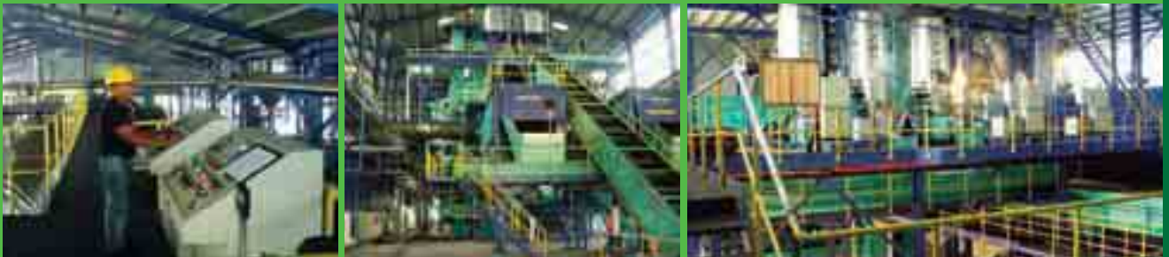
Automated mill processes at Genting Indah Oil Mill - process synchronisation &amp; automation system
