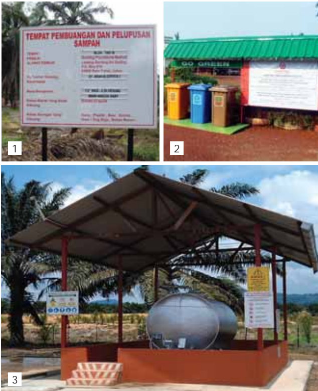
1-2. Good practices for environmental stewardship 3. Bunding for pollution control
