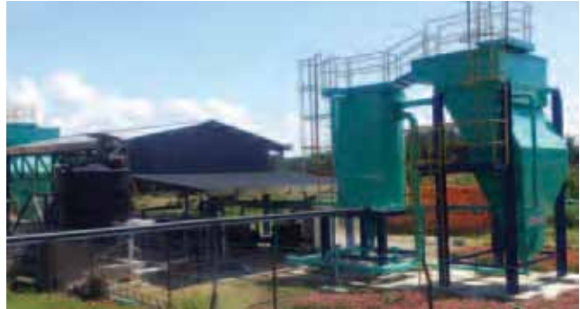
Membrane bioreactor plant treats palm oil mill effluents to ensure biochemical oxygen demand are at permissible levels.
