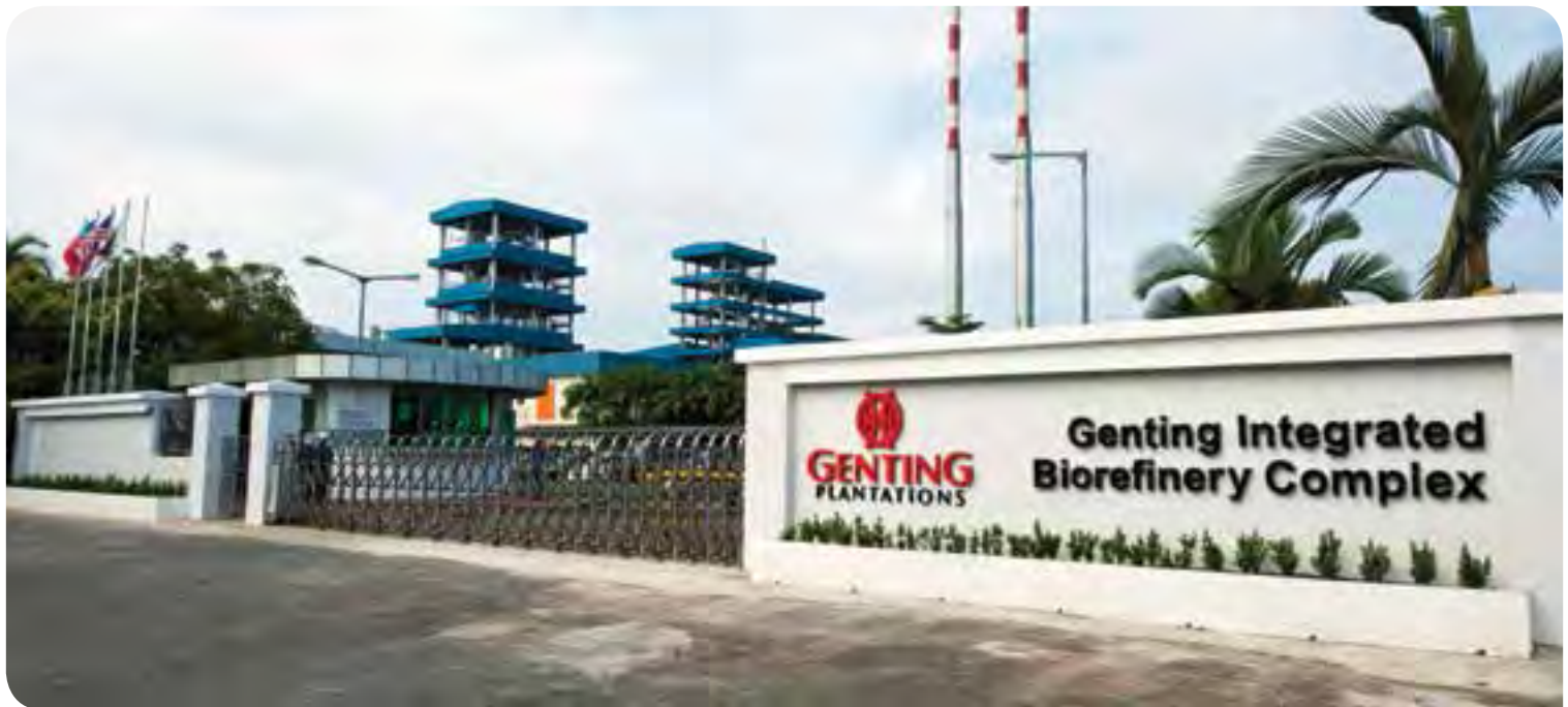
Genting Integrated Biorefinery Complex, Sabah
