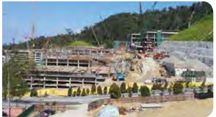
Genting Premium Outlets under construction
