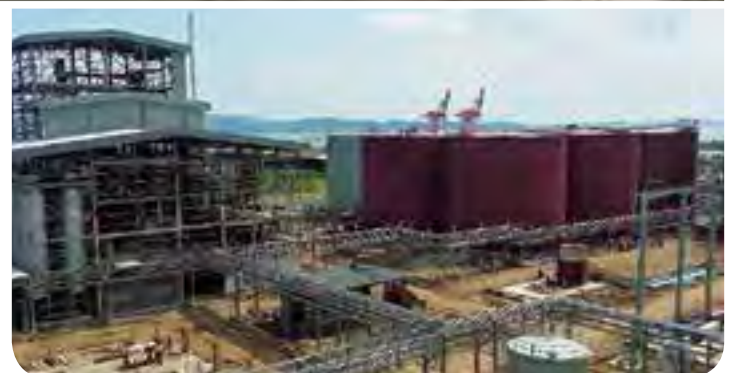
Refinery under construction
