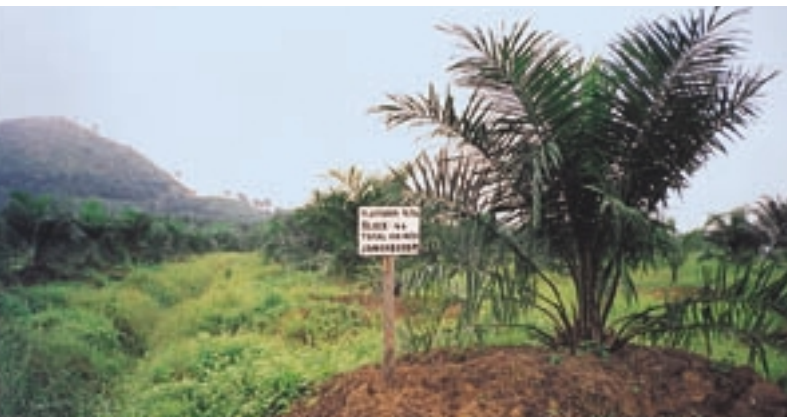
Palms planted on raised platforms - part of the rehabilitation works on the flood-damaged areas in Tenegang, Sabah.
