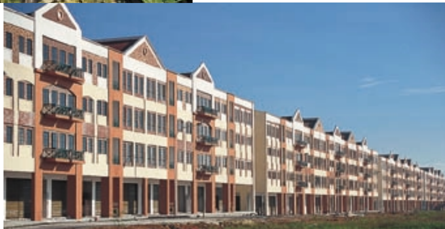
Completed 4-storey shop offices in Indahpura.
