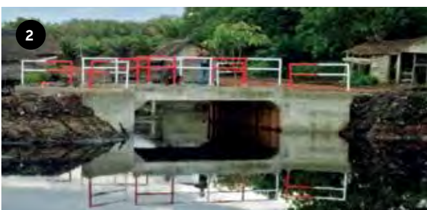
Flood mitigation projects implemented included the construction of 1. Concrete bridge 2. Box culvert bridge 3. Bund
