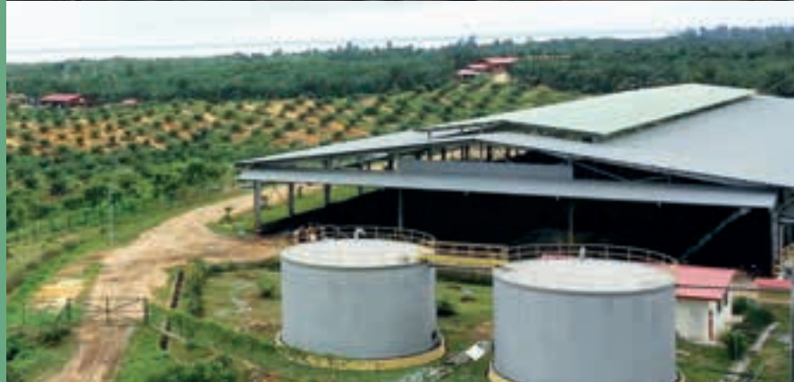
Compost plant at Genting Jambongan Oil Mill.
