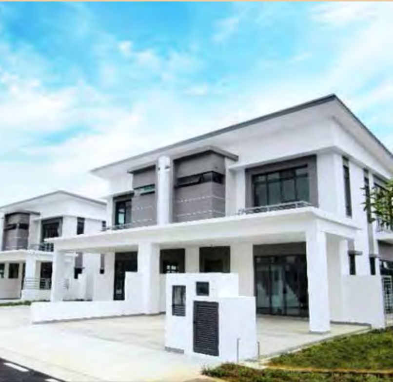
Raintree Residences (Phase 2) at Genting Indahpura – construction completed ahead of schedule
