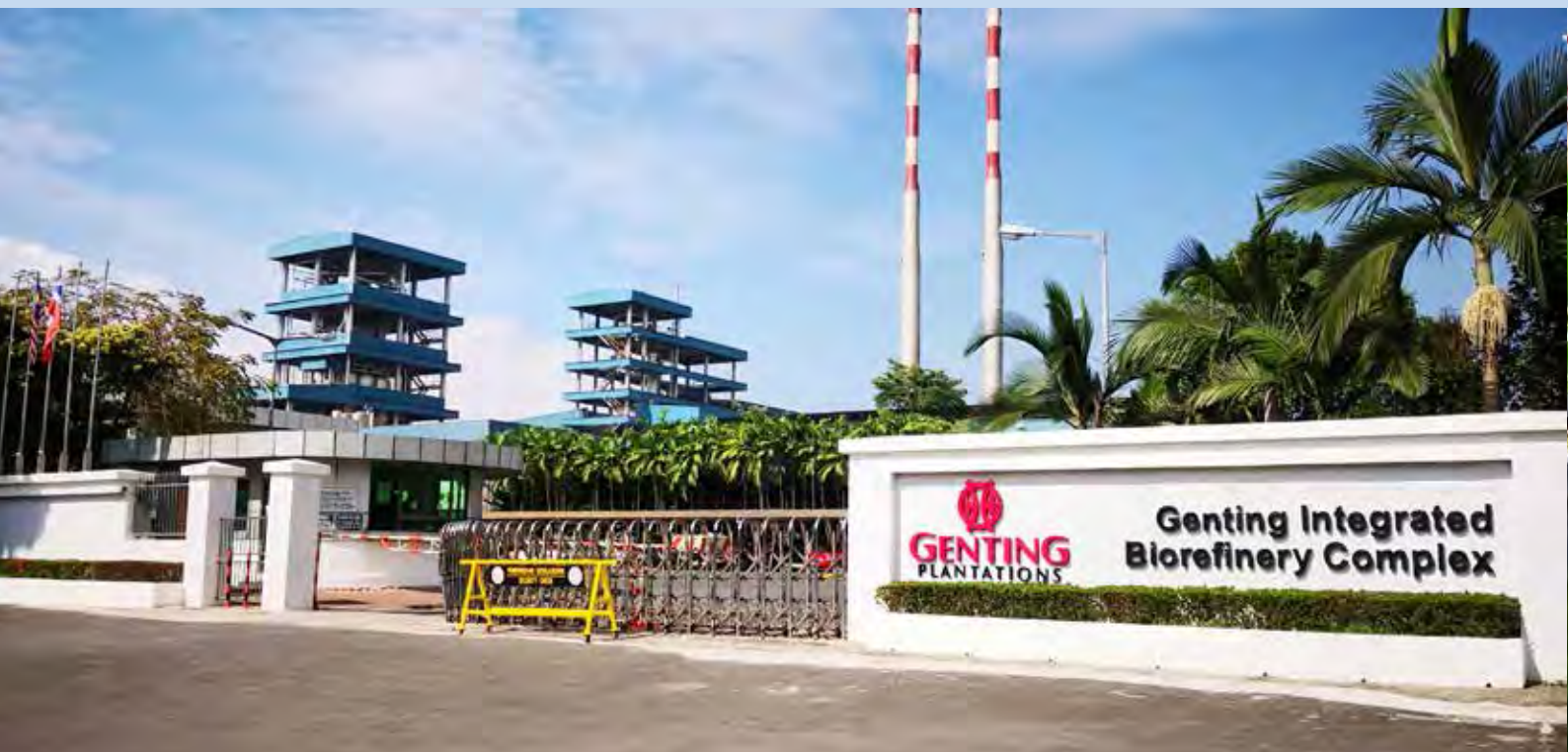
Genting Integrated Biorefinery Complex at POIC Lahad Datu, Sabah
