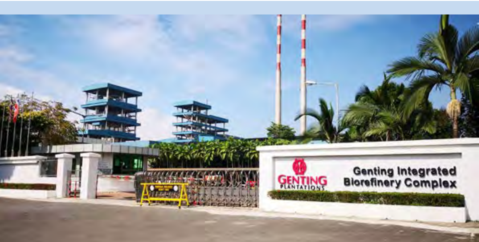
Genting Integrated Biorefinery Complex at POIC Lahad Datu, Sabah
